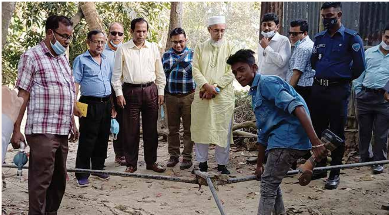
Inspection of Illegal Gas Pipeline Removal Activities
