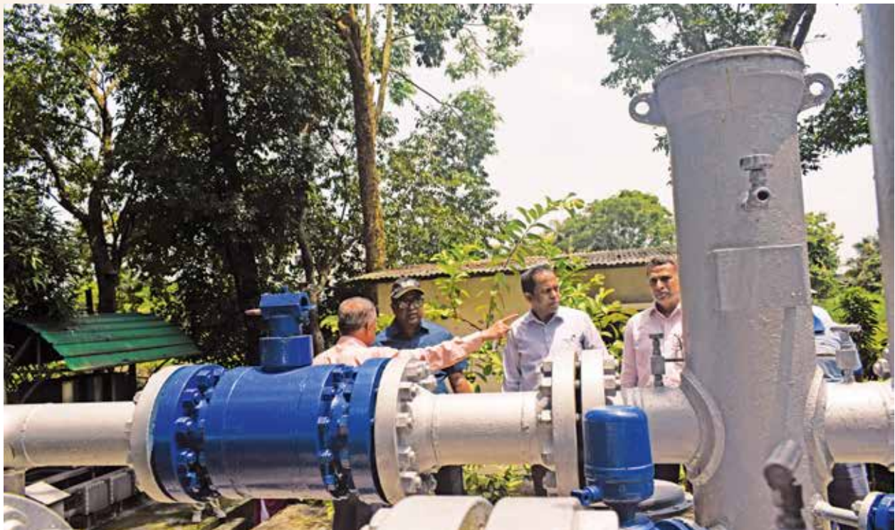
Visit of Gouripur Metering Station of BGDCL by Hon'ble Chairman, Petrobangla
