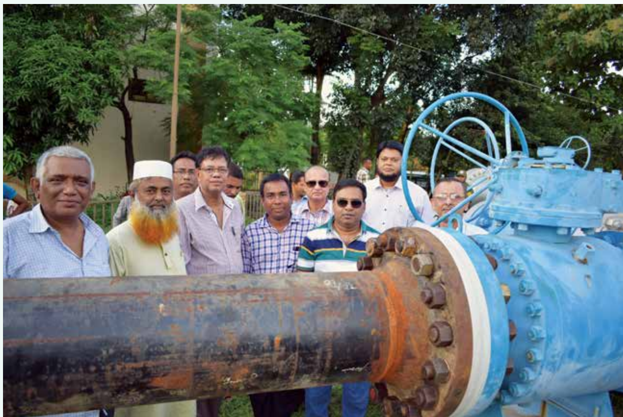
Inauguration of Gas Supply to Ashuganj Fertilizer through newly constructed pipeline.
